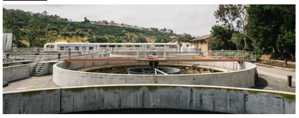
Guarding the environment and creating new water supplies requires among the most advanced treatment facilities in the State. SOCWA's three primary treatment facilities can treat upwards of 26 million gallons of wastewater per day. Historically, about half of this water is treated for recycled water use. The balance is treated and discharged miles off our coast through two ocean outfalls.
